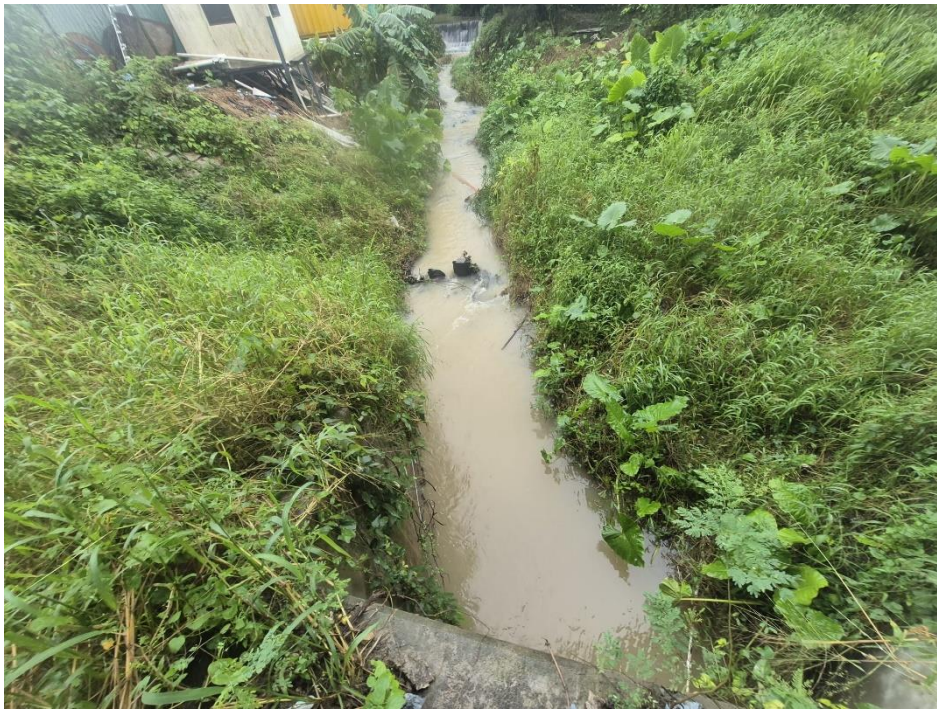
Photo 3a (Taken at C1 Station on 31 July 2026)
