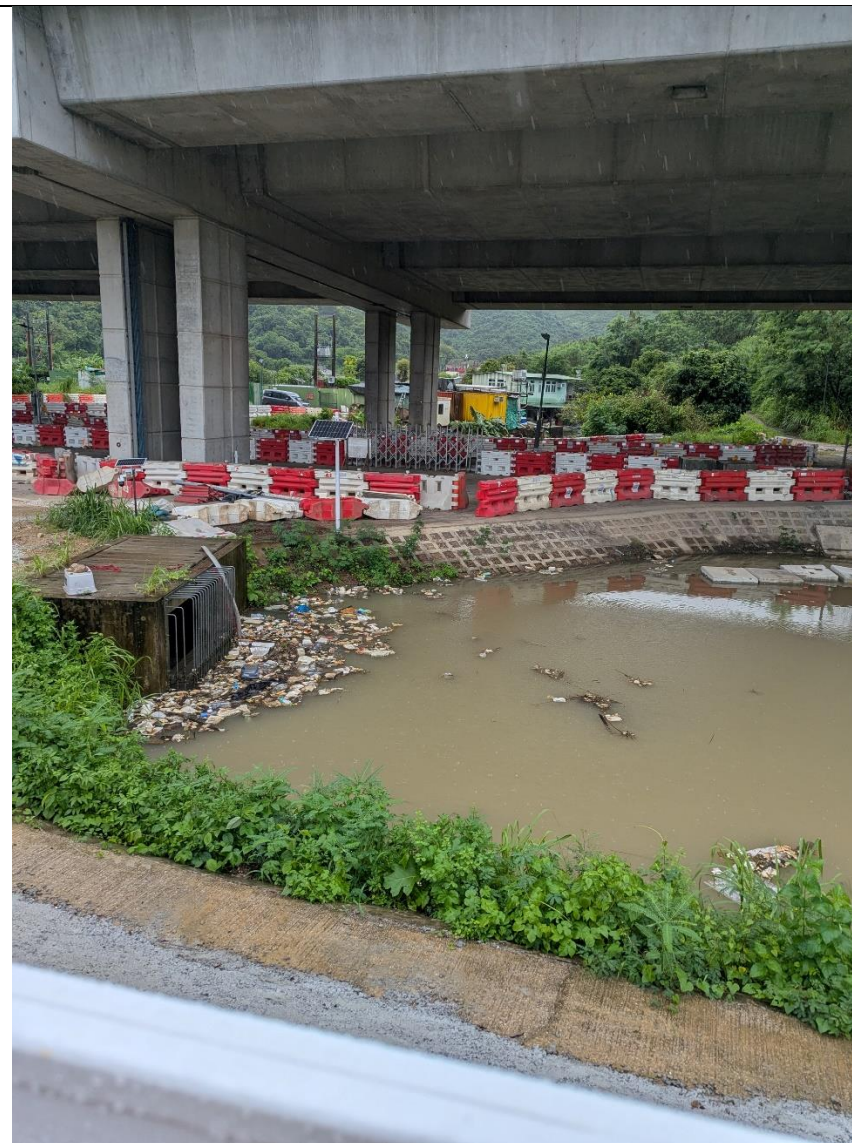
Photo 5 (Taken at the Sub-Channel under Kong Sham Western Highway on 31 July 2026)
