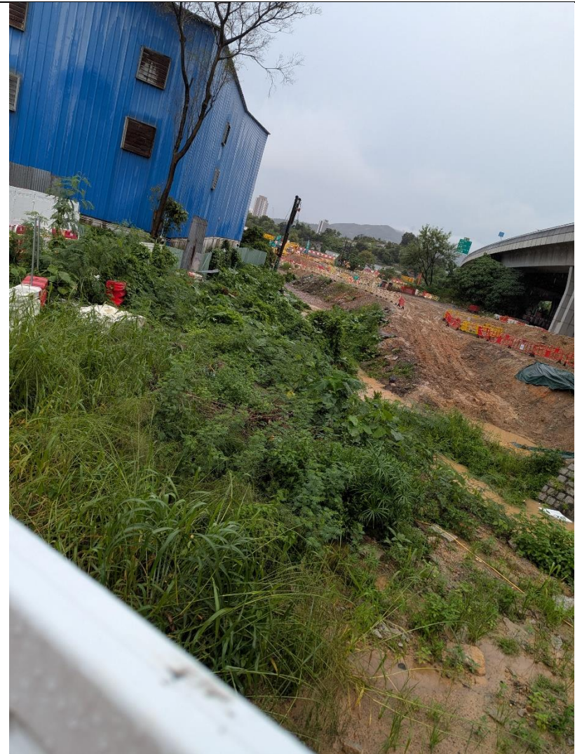
Photo 7 (Taken at the site boundary between the DSD construction site and CEDD construction site on 31 July 2026)
