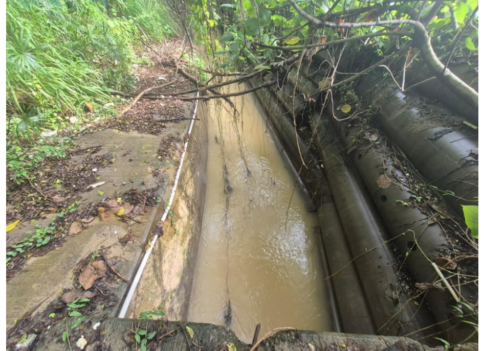
Photo 2b (Taken at M1 Station on 17 July 2026)
