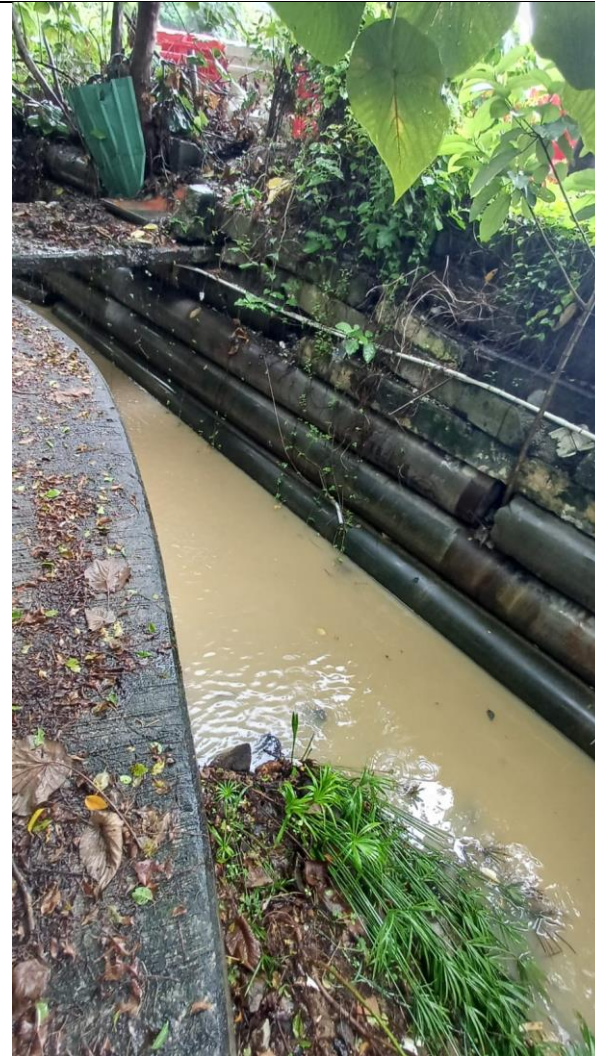
Photo 1b (Taken at M1 Station on 06 July 2026)
