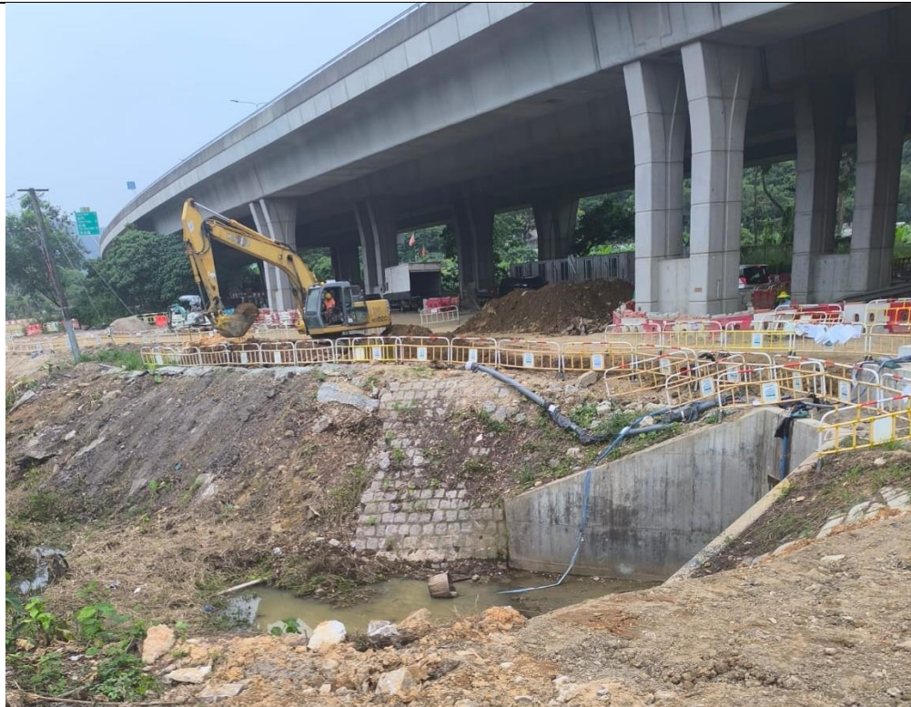
Photo 6 (Taken at the downstream of C1 near Kong Sham Western Highway on 12 June 2026)
