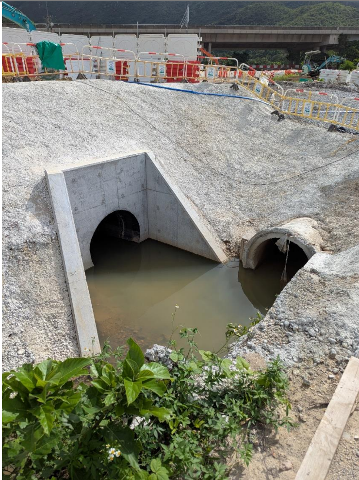
Photo 4 (Taken at CEDD Construction site on 20 June 2026)
