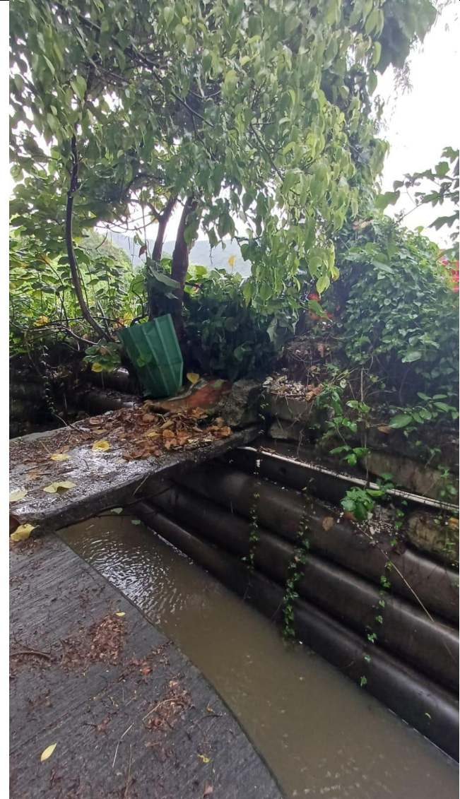
Photo 2b (Taken at M1 Station on 15 June 2026)
