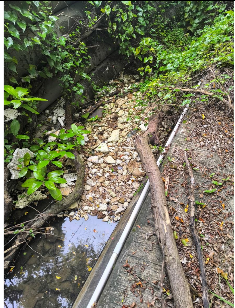
Photo 5 (Taken at the upstream of Monitoring station M1 on 12 June 2026)
