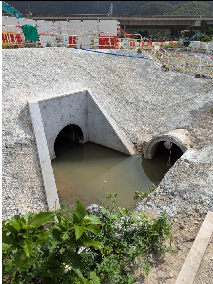
Photo 4 (Taken at CEDD Construction site on 20 June 2026)
