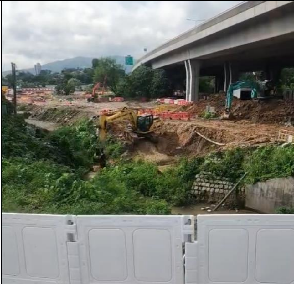
Photo 8 (Taken at the site boundary between the DSD construction site and CEDD construction site on 29 July 2026)
