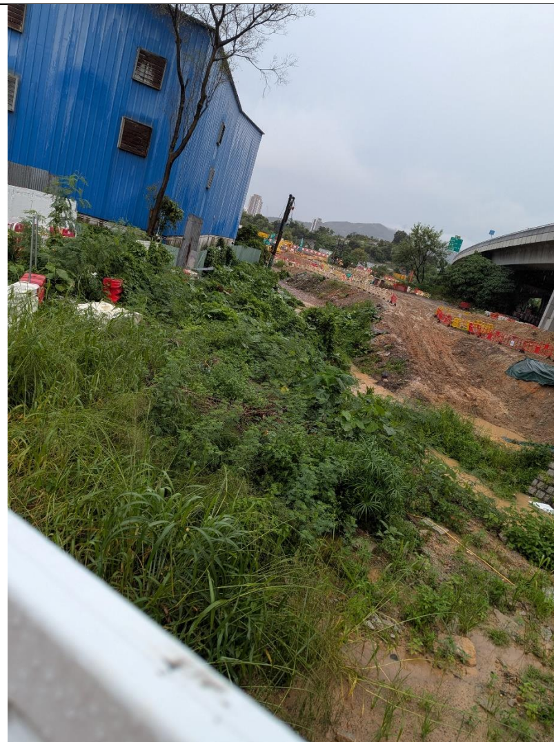
Photo 7 (Taken at the site boundary between the DSD construction site and CEDD construction site on 31 July 2026)
