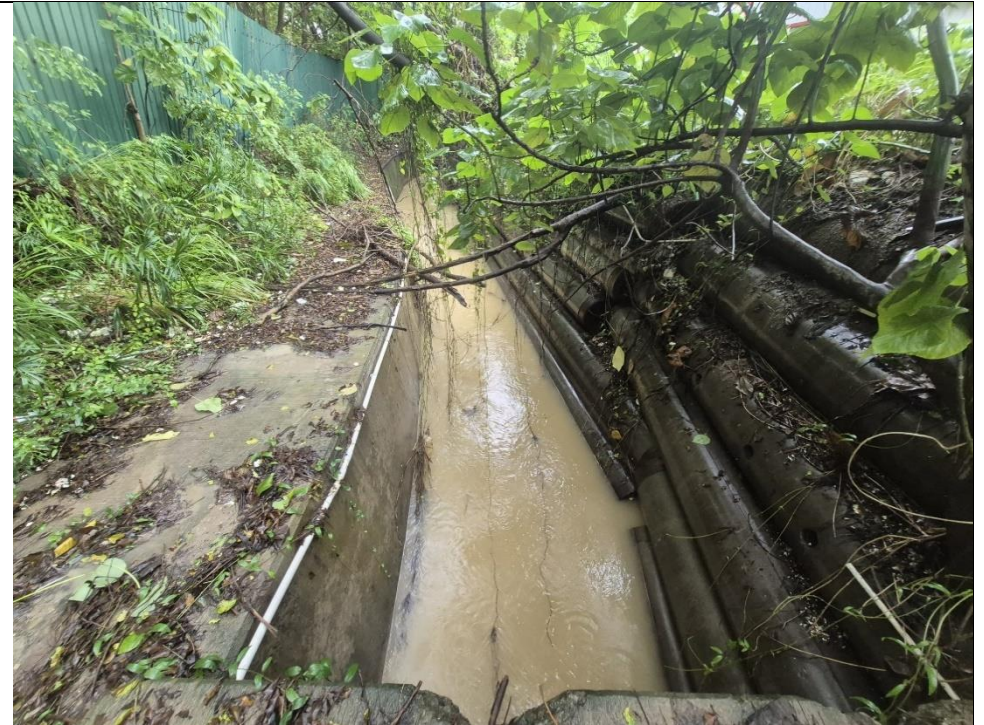
Photo 3b (Taken at M1 Station on 31 July 2026)
