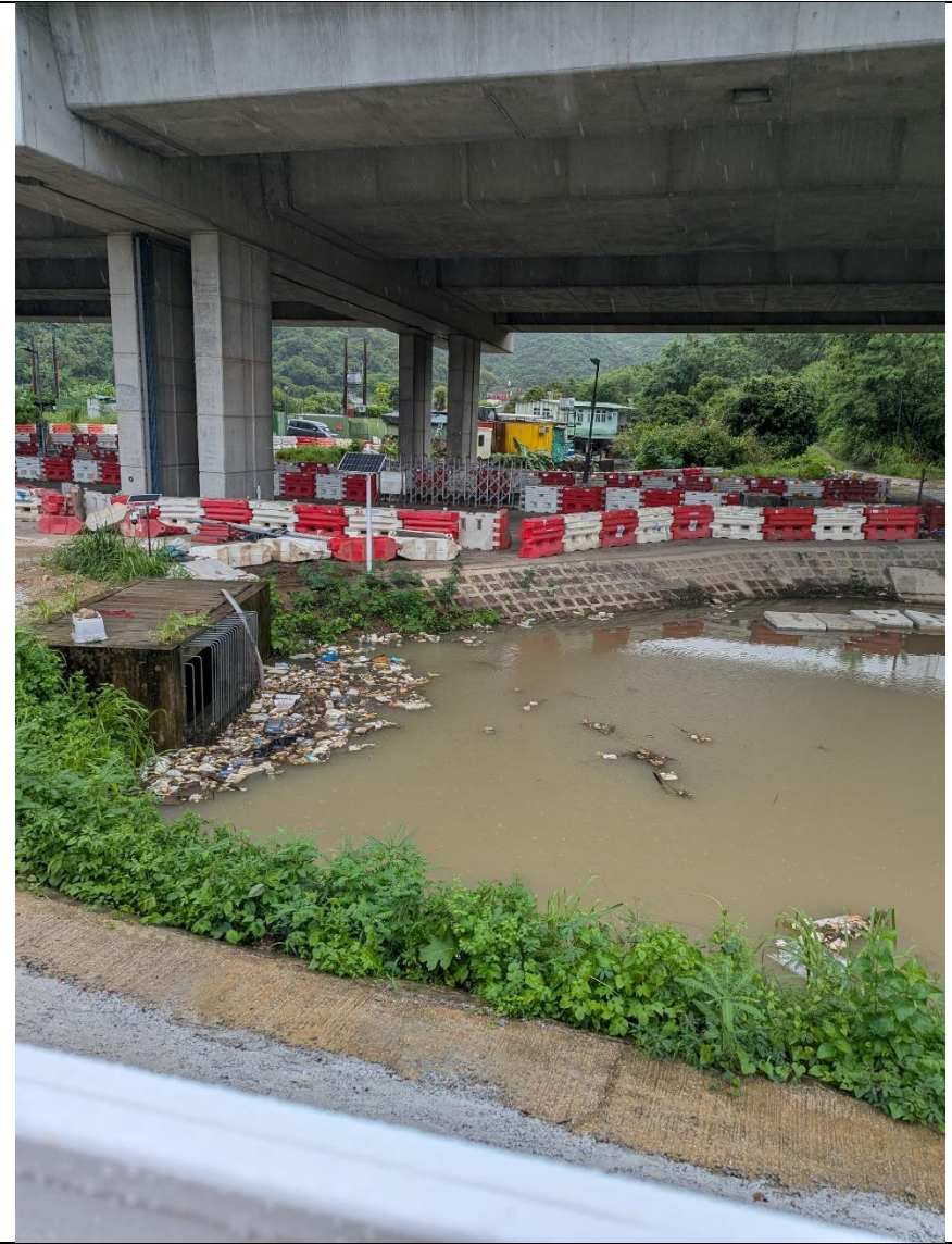
Photo 5 (Taken at the Sub-Channel under Kong Sham Western Highway on 31 July 2026)
